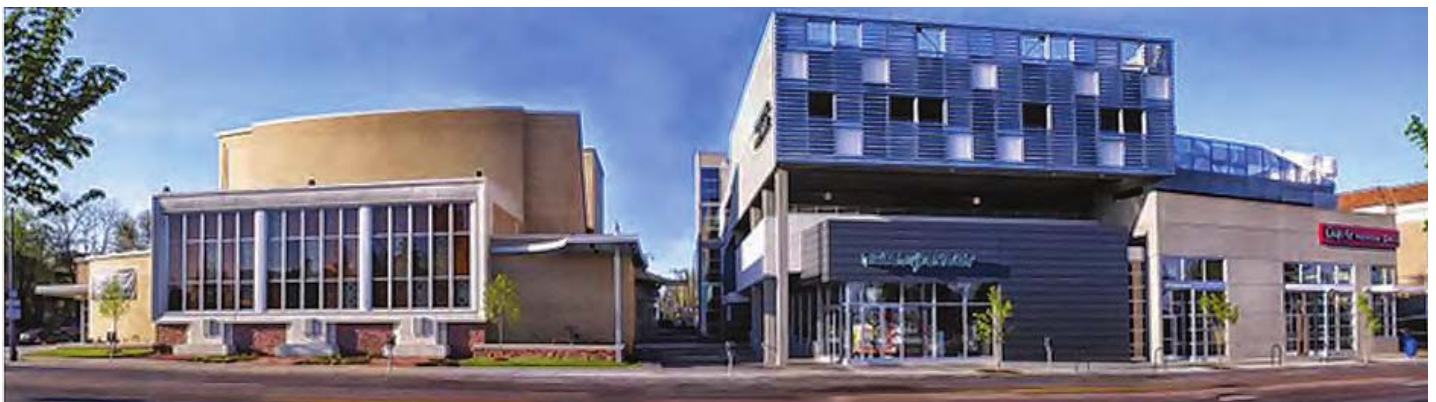
One strategy for the area is to redevelop outmoded retail for other uses, such as employment centers, civic and cultural amenities, residential and/or mixed-use areas. Photo credit: ULI Oklahoma.
